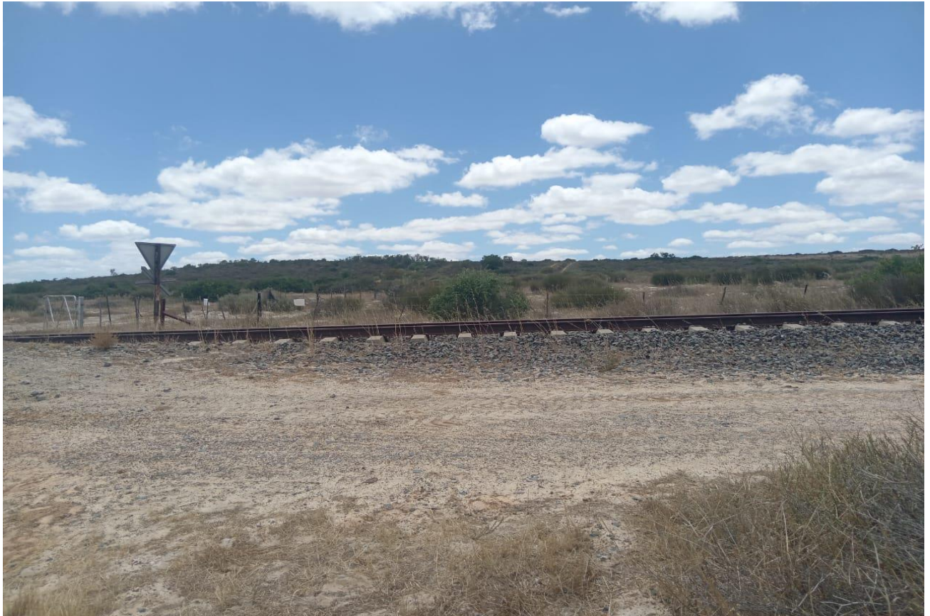
Figure 4: View of the railway line that traverses through the farm.
