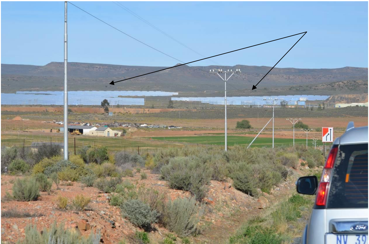
Figure 16: Existing Touws River Solar Farm
