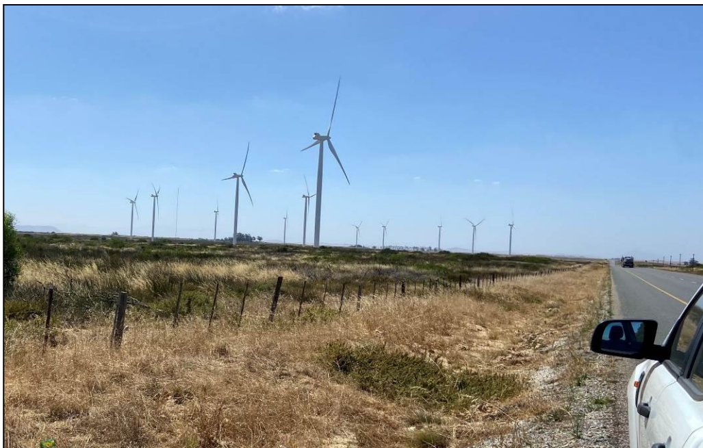
Figure 19: Existing Renewable Power Infrastructure
