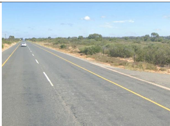
Sight Distance to the right at the Existing Access along the R45
