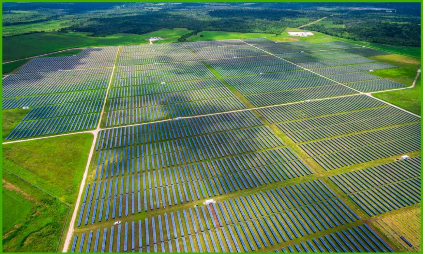
Figure 1: Picture of solar PV plant development
