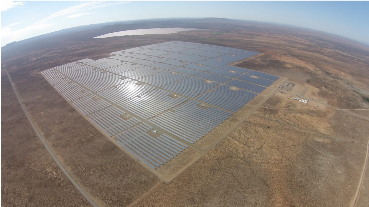
Figure 3: Photo showing the aerial view of the PV facility
